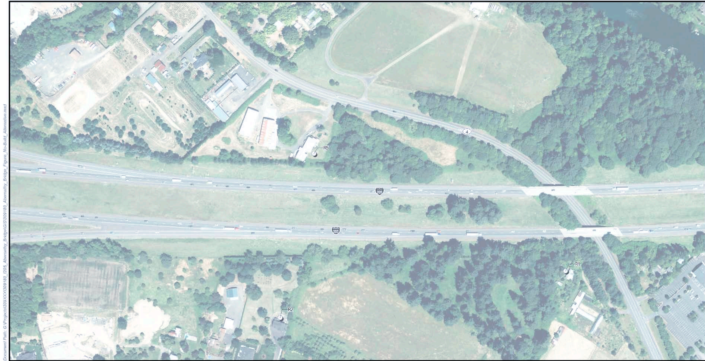
Figure 4. Existing Conditions/No Build Alternative
