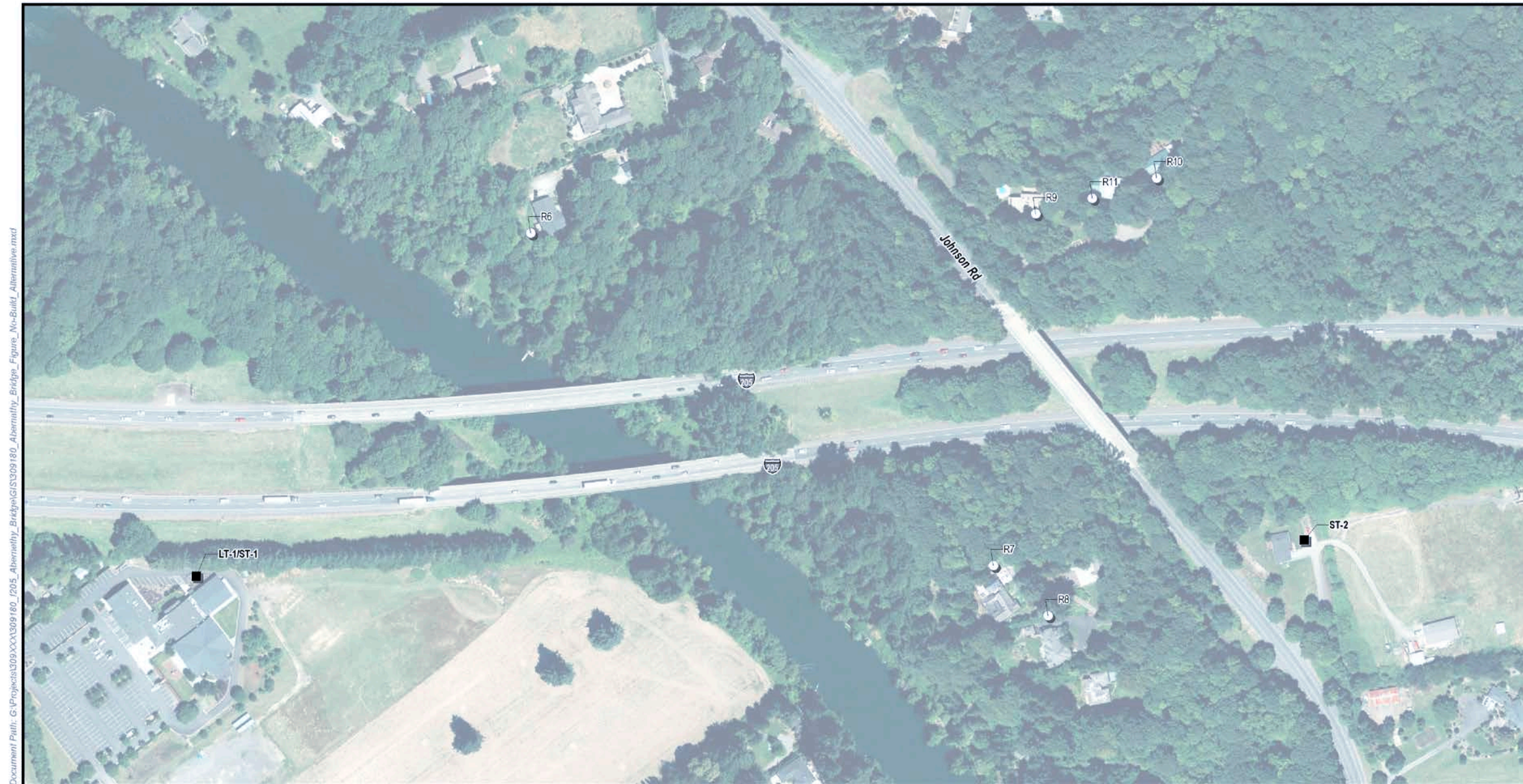
Figure 5. Existing Conditions/No Build Alternative
