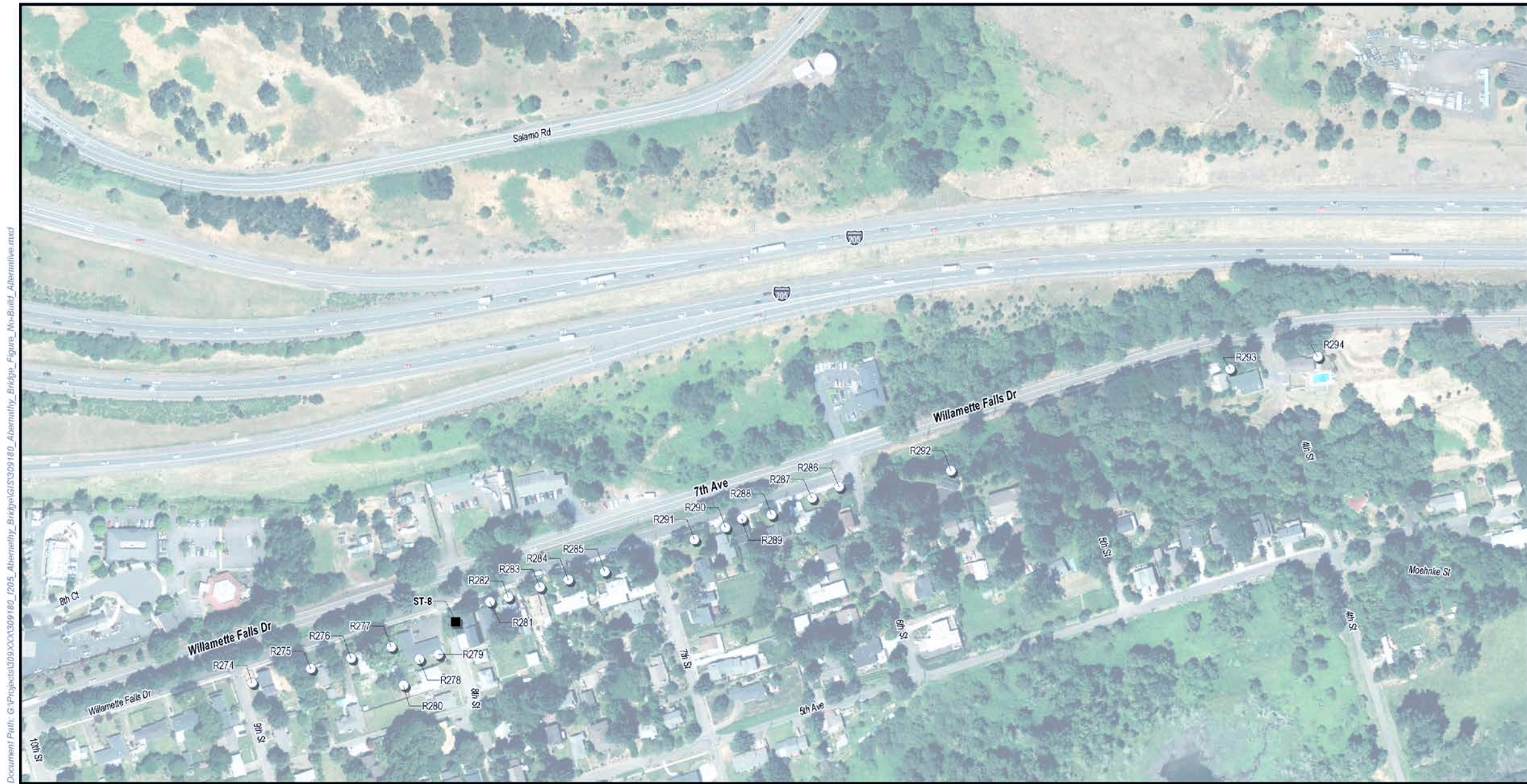
Figure 10. Existing Conditions/No Build Alternative
