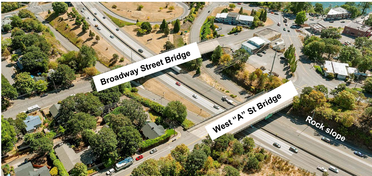
Figure 21. Photograph of Broadway Bridge (to be removed), West A Street Bridge (to be replaced), and the Rock Slope area (to be cut back)
