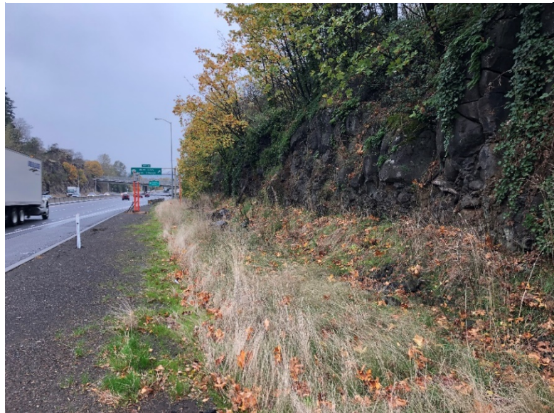
Figure 20. View of an Existing Project Rock Cut Area
